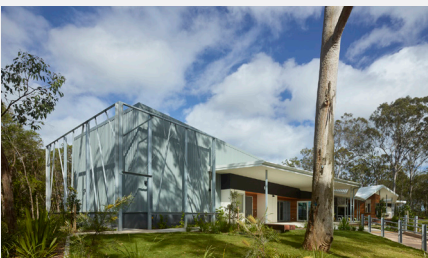
Kimberley College, Art & Library Buildings, Carbrook
