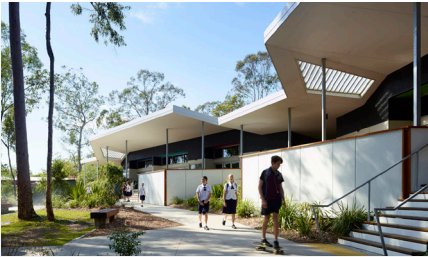
Kimberley College, Year 7 Building, Carbrook
